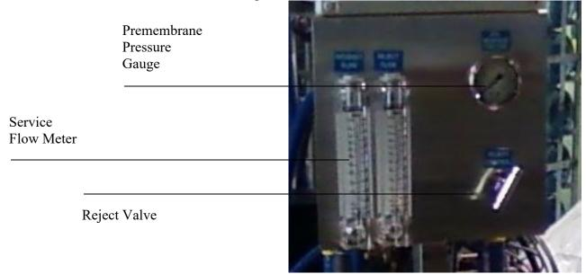
B. Check the service water quality on the meter on ROC Controller
